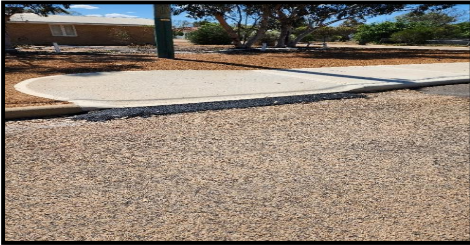
Repairs to footpath on Gamble Street allowing easy access for pedestrians.
