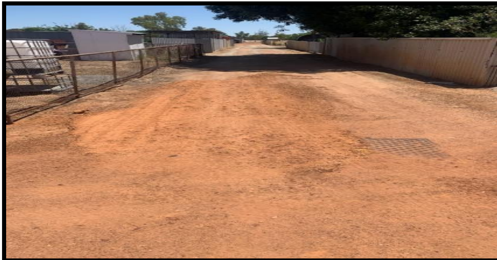
Gravel was used to fill in the ruts in the laneways.
